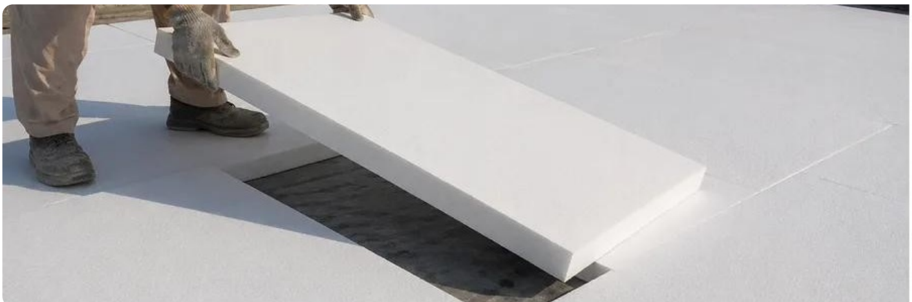
EPS sheets being laid on a roof ahead of the protective screed.
